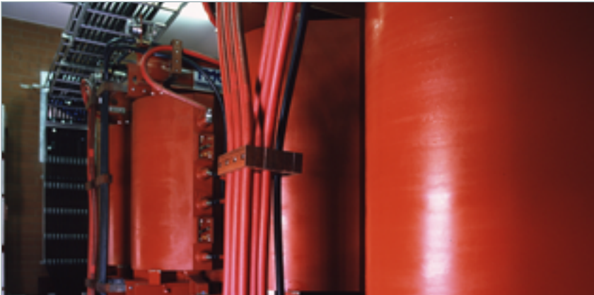
2.5MVA power transformer installation
