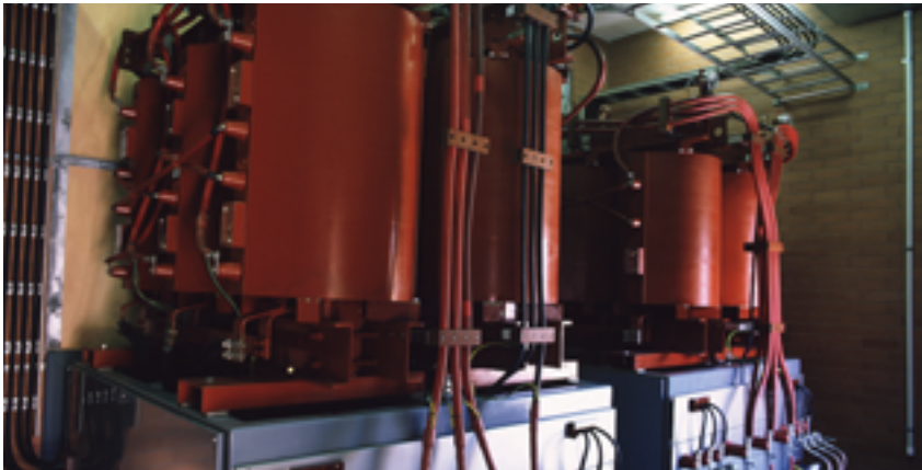
2.5MVA power transformer installation
